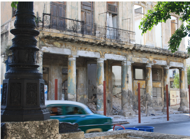
Photo 8. Dilapidated Old Havana Source: S. Kaczmarek (February 2014)
