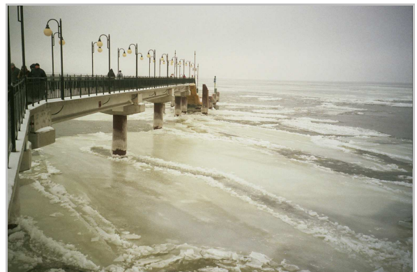
Photo 8. Floe cut by the pier pillars (Międzyzdroje, 30 th December 2010)
