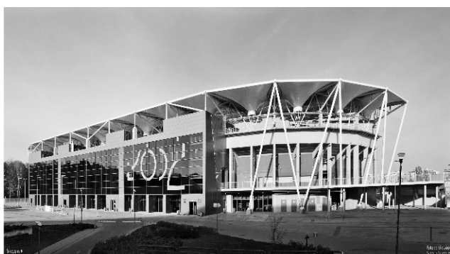
Photo 3. ŁKS City stadium (under construction) Source: http://fotopolska.eu/stadiony
