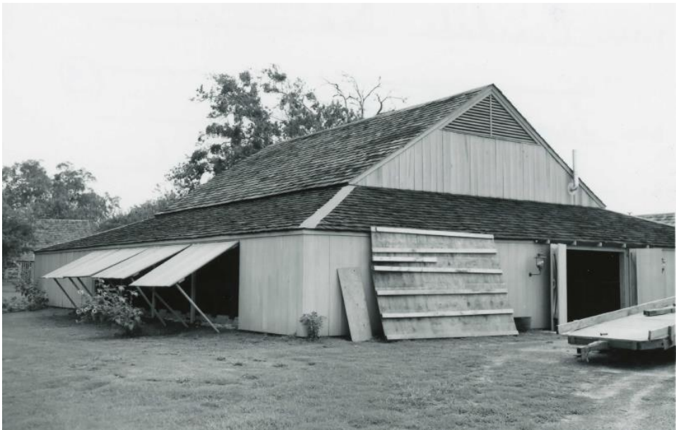
Figure 4: The Winedale theater-barn as it appeared in 1970. Wayne Bell papers, University of Texas at Austin. Wayne Bell’s surveys determined that the beams had been recycled from a cotton gin and cotton press. The beams were likely carved by enslaved Black laborers
