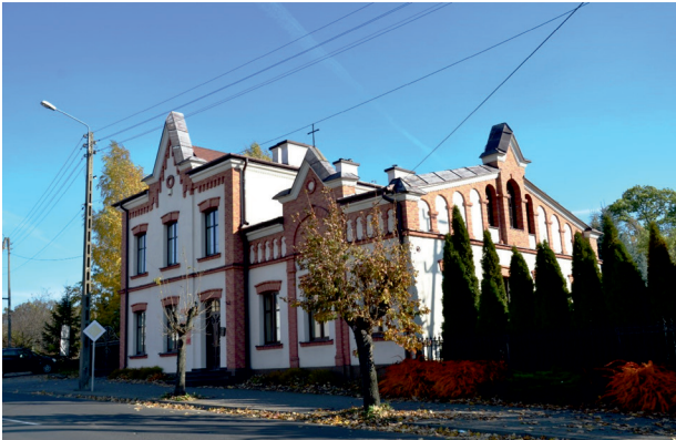
Photo 3. A former parish house in Brzeziny
