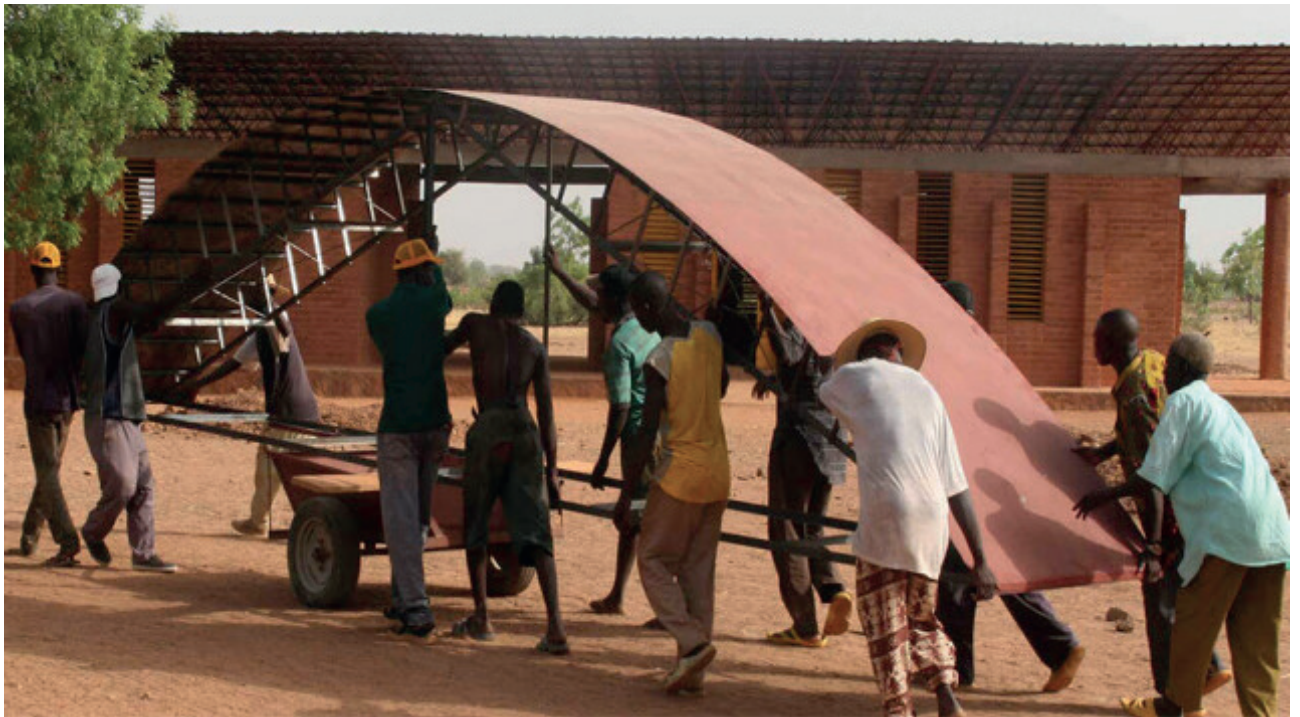
Illustration 2. Formwork for clay brick ceiling, School Extension. Photo by Francis Kéré
