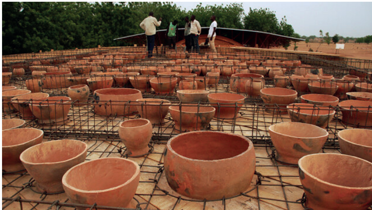
Illustration 4. Gando School Library, formwork concrete ceiling. Photo by Kéré Architecture GmbH
