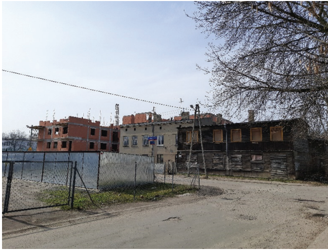
Figure 2. Diverse architecture on Młynarska Street
