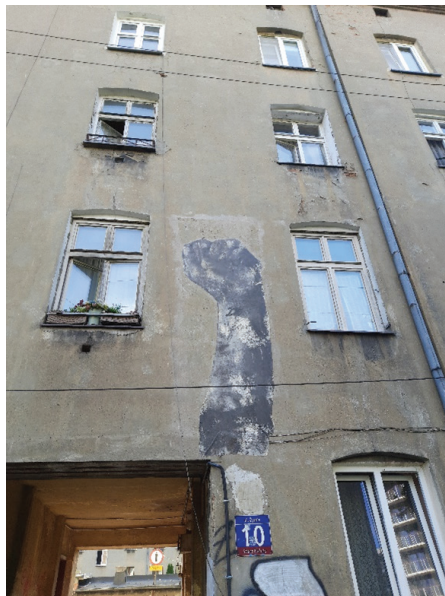
Figure 3. Work on Żytnia Street showing the tattoo of one of the residents
