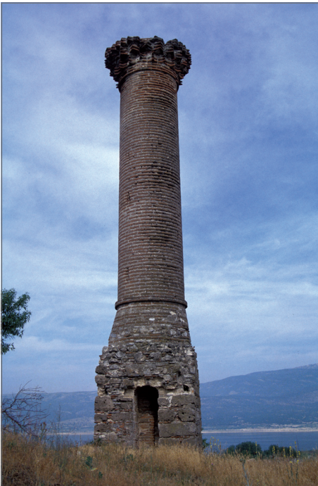
Fig. 4. The remnants of the minaret (15 th cent.) (Peter Soustal, 1993)
