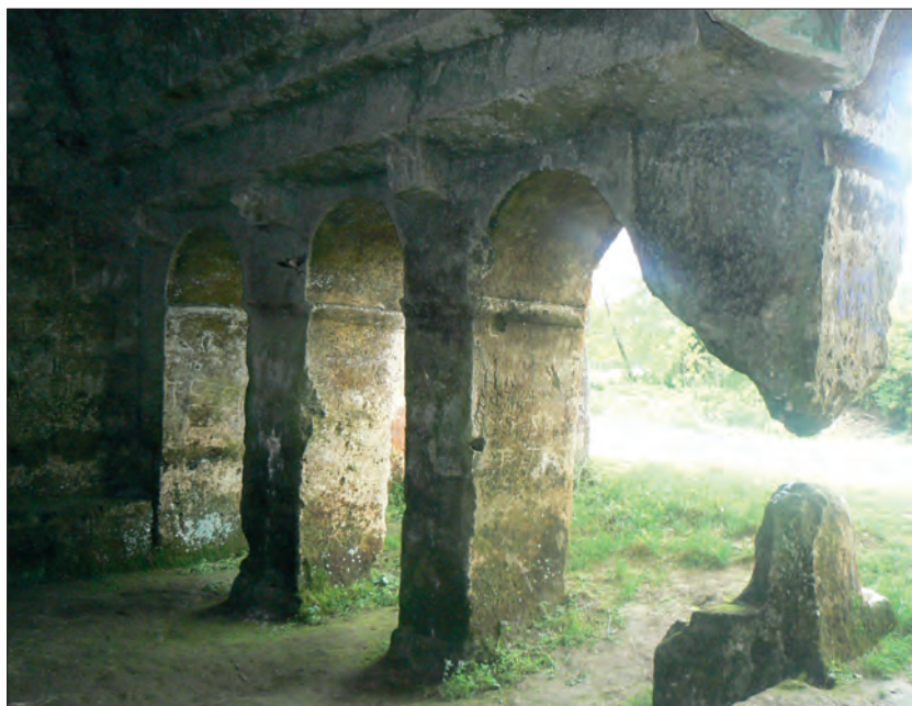
Fig. 18. The two “columns” between the central and left (north) naves.
