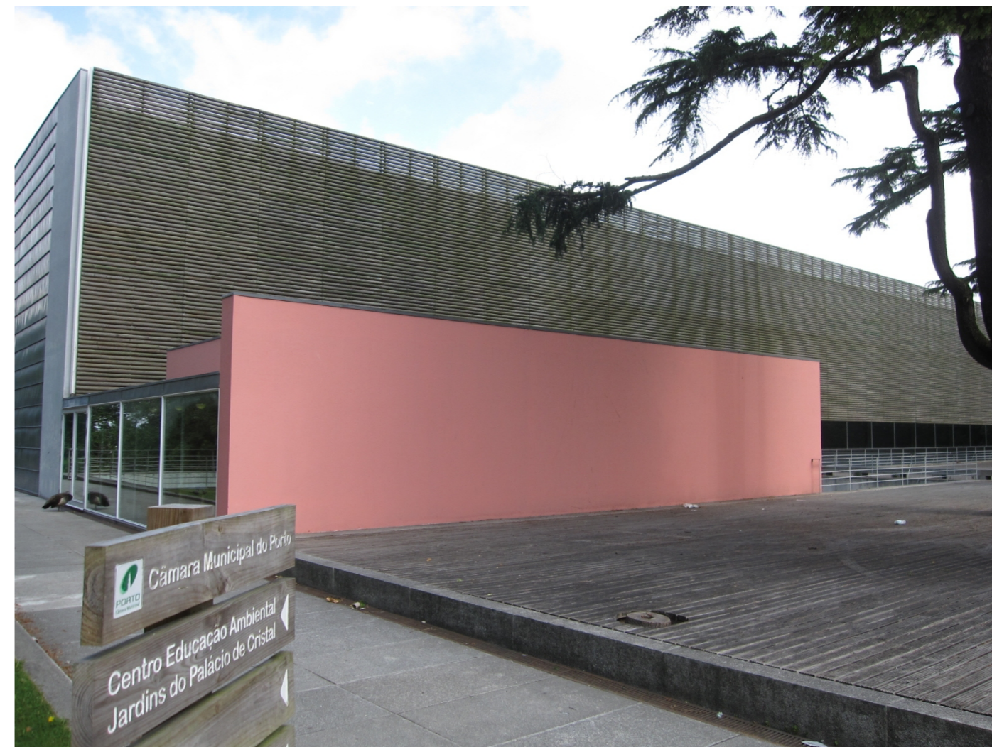
Figure 2. The main façade of the Almeida Garrett Library.
