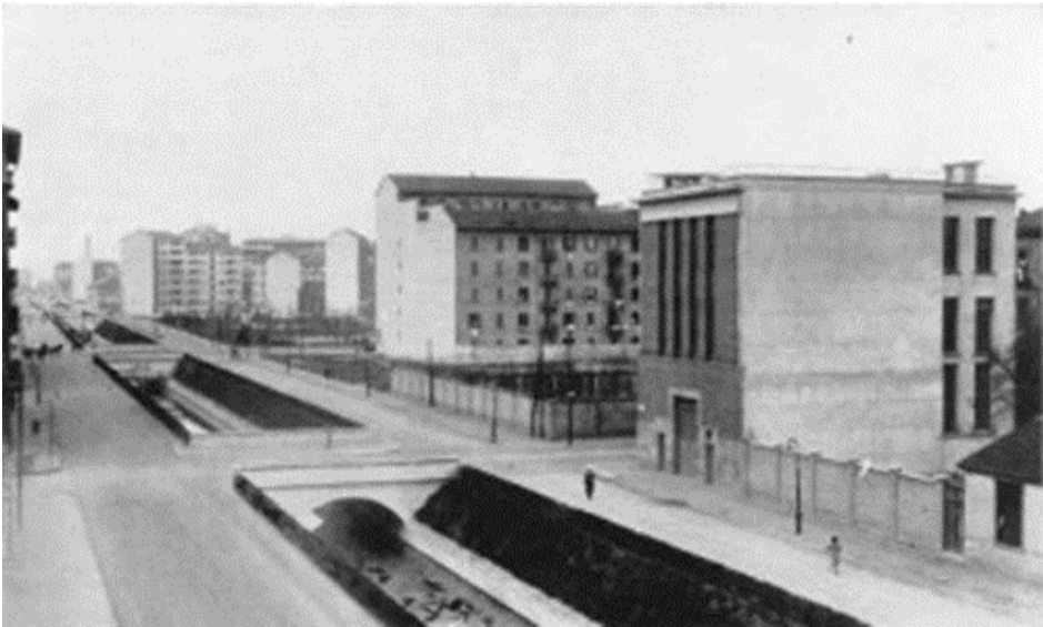
Fig. 3. The first phase of the reconstruction of the Olona riverbed until its filling, 1930s. Source: author's archive.
