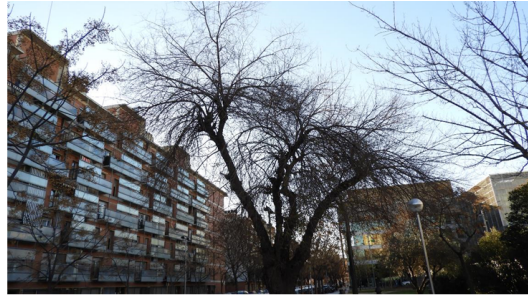
Built blocs in stages 1 to 3
