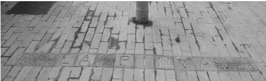
Fig. 30. Panots – the first intervention of the 13 planned.
