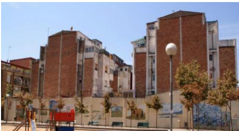
Fig. 23. A view of the Party Walls in 2001.
