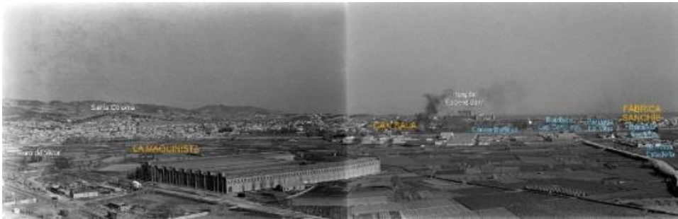
Fig. 3. General view of the territory in the first half of the 20 th century. In the foreground, the factory of the Terrestrial and Maritime Machinist. The rural character of the territory can be seen.
