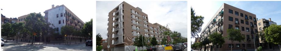
Fig. 12–16. Plan of the different relocation phases. Source: Registre de Planejament Urbanístic de Barcelona. New housing blocks built in the relocation plan.
