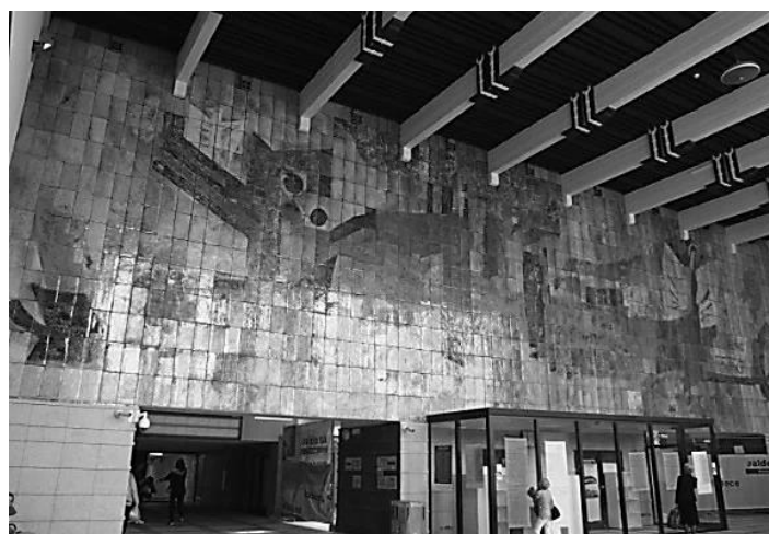
Fig. 6. Gliwice, Railway Station , Zygmunt Lis, Witold Bulik, Bolesław Książek, 1967. Photo by Bożena Kostuch, 2016.
