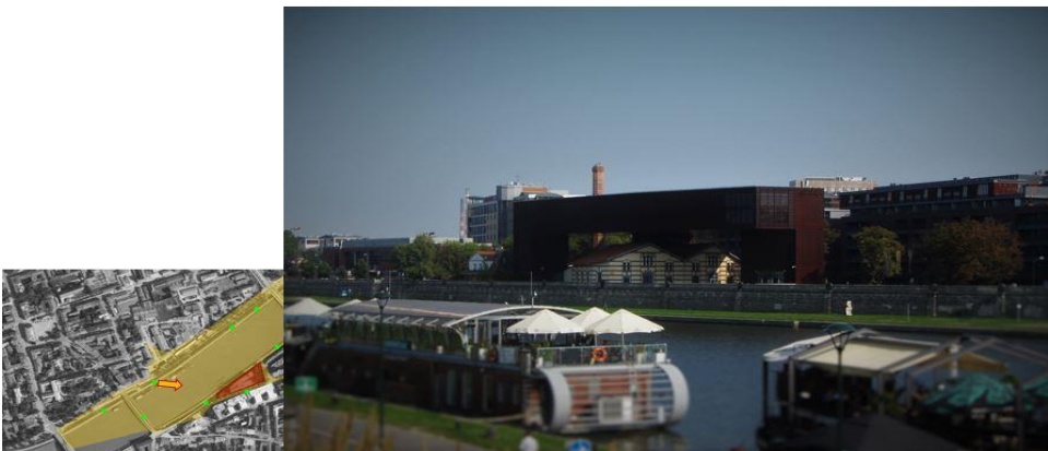
Fig.6. View of the building Cricoteka from across the Vistula Boulevard. Photo by Ewa M. Romaniak.
