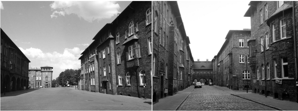
Fig. 3, 4. Post office building and familoki in Nikiszowiec. Photo by Ewa Waryś, 2016.
