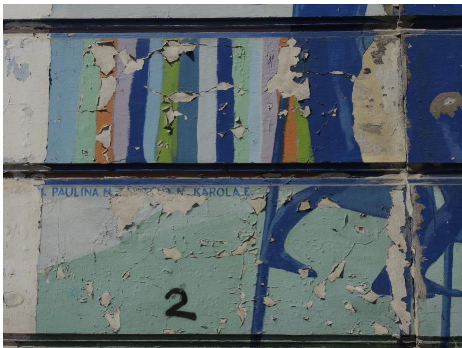
Fig. 6. Linas Damarackas, Stilters , detail, 2008, 37 Stalowa Street, Warsaw, the flaking paint layer on the mural. Photo by Tytus Sawicki (2018)
