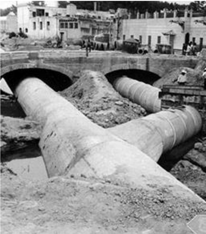
Fig. 8. Piping of the “San Francisco” river, prior to its burying and the construction of the boulevard “Héroes del 5 de Mayo” (Puebla General Municipal Archive, 1960 ca). Photo: authors’ archive.
