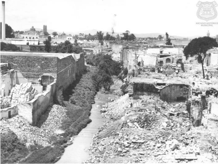
Fig. 7. General view of the “San Francisco” river during the demolition of houses on the banks for the future construction of the “Héroes del 5 de Mayo” boulevard (Puebla General Municipal Archive, 1957 ca). Photo: authors’ archive.
