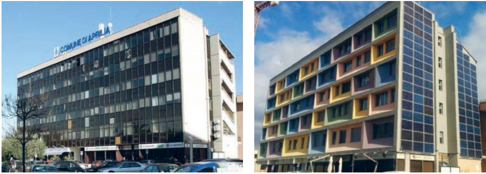
Fig. 6. The Town Hall, before and after the works
