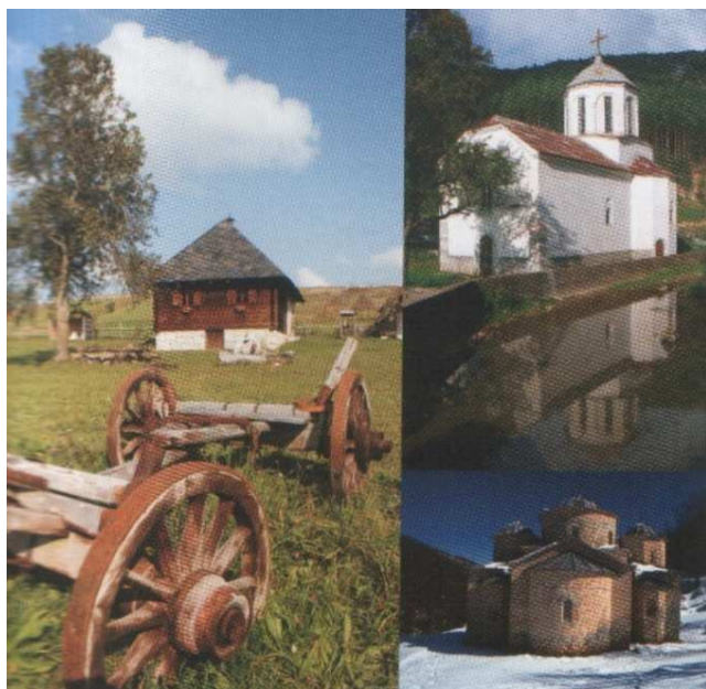
Photo 16. Outside Nova Varoš, South-Western Serbia. Almost deserted village household and two monastery Orthodox Church buildings in a peaceful and quiet Serbian landscape Source: Three Unique Days in Nova Varoš , USAID (2007)
