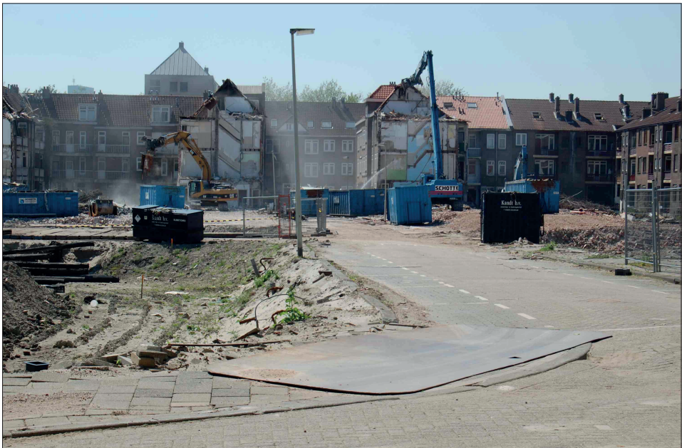
Fig. 2. Demolition in Nieuw Crooswijk (2007) Source: own
