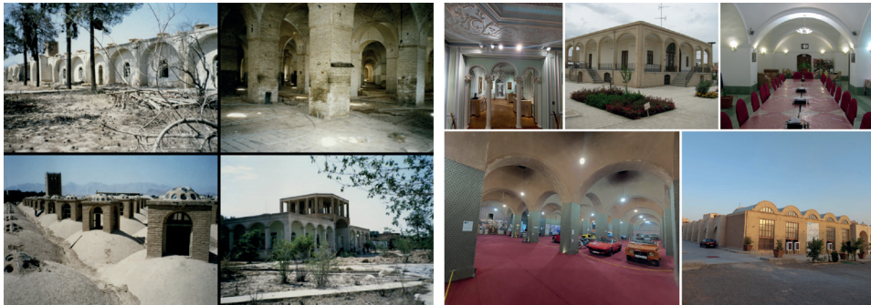
Fig. 4. Textile factories before and after revitalisation in Yazd
