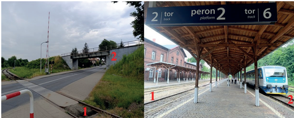
Fig. 3. Photos of the tracks in stations Gluchołazy-Center (left) and Gluchołazy (right) Source: own work (2025).
