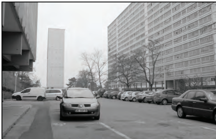
Fig. 6. Image of the original buildings of La Duchère Source: Paul Stouten
