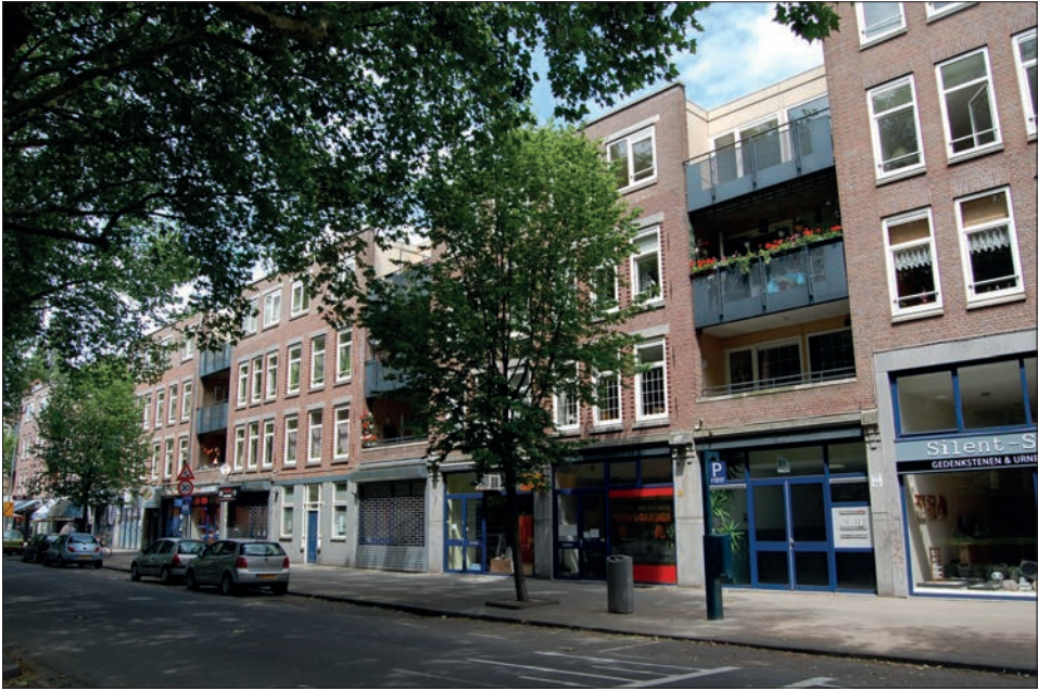
Fig. 5. Saved from demolition Source: own
