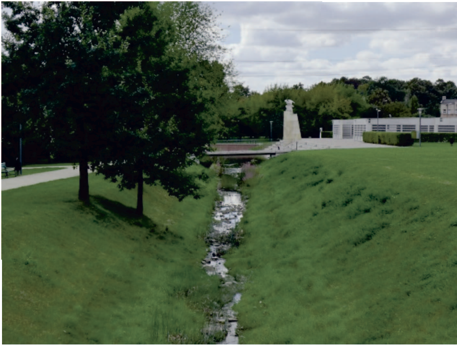
Fig. 4. Straight, regulated part of the river in the park Source: photograph by E. Kobojek
