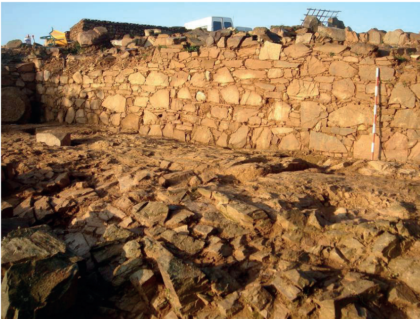
Fig. 12. The foundation in stone masonry of western wall of the room 7 (Can Tacó team).
