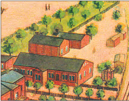
Fig. 10. The ice house at the Konsum building. A view from the north-east as of the period between 1897 and 1899, source: Zjednoczone zakłady... (fragm.).
