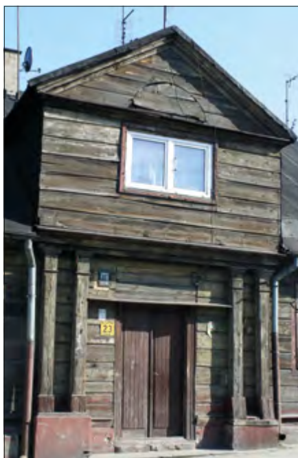
Fig. 3. Pilasters flanking the entrance and ‘supporting’ the mansard window of the house at 23 1 Maja Street (source: the collection of the D.O.M. foundation).
