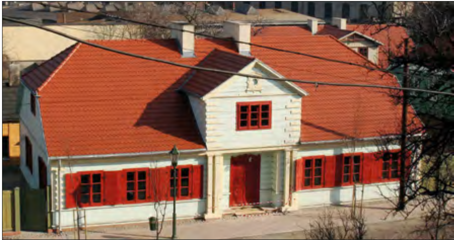
Fig. 2. The Weaver's House at 5 Narutowicza Street, as seen from Rembowskiego Street (source: the collection of the D.O.M. foundation).
