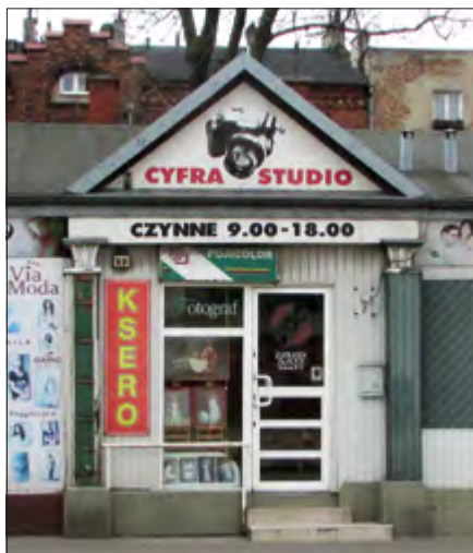
Fig. 17. The preserved column capitals and the triangular gable added to the elevation of the building at 38 Długa Street (source: the collection of the D.O.M. foundation).
