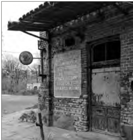
Fig. 1. A fragment of the buildings located at the main entrance in Kilińskiego Street – Alicja Piotrowska's private archive.
