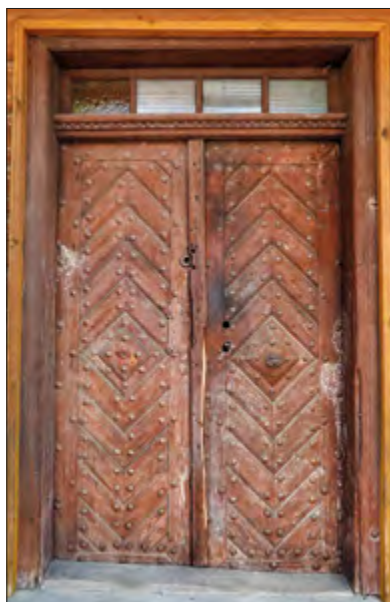
Fig. 7. A diamond-boarded door, at 29 Narutowicza Street (source: the collection of the D.O.M. foundation).
