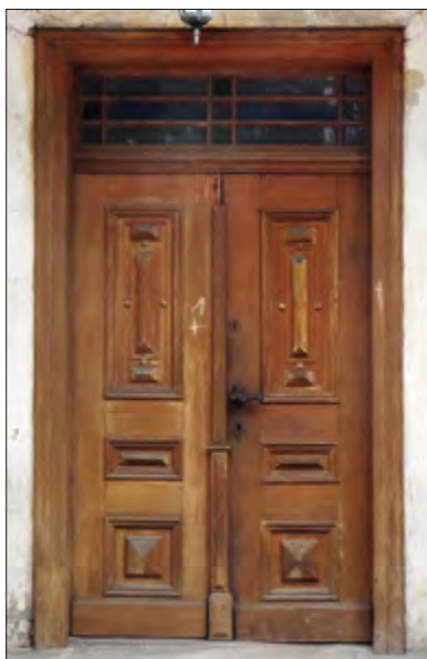
Fig. 6. A frame-and-panel door at 7 Narutowicza Street (source: the collection of the D.O.M. foundation).
