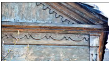
Fig. 4. Decorative slats on the façade of the building at 16 Dąbrowskiego Street (photograph by P. Trzeźwiński).
