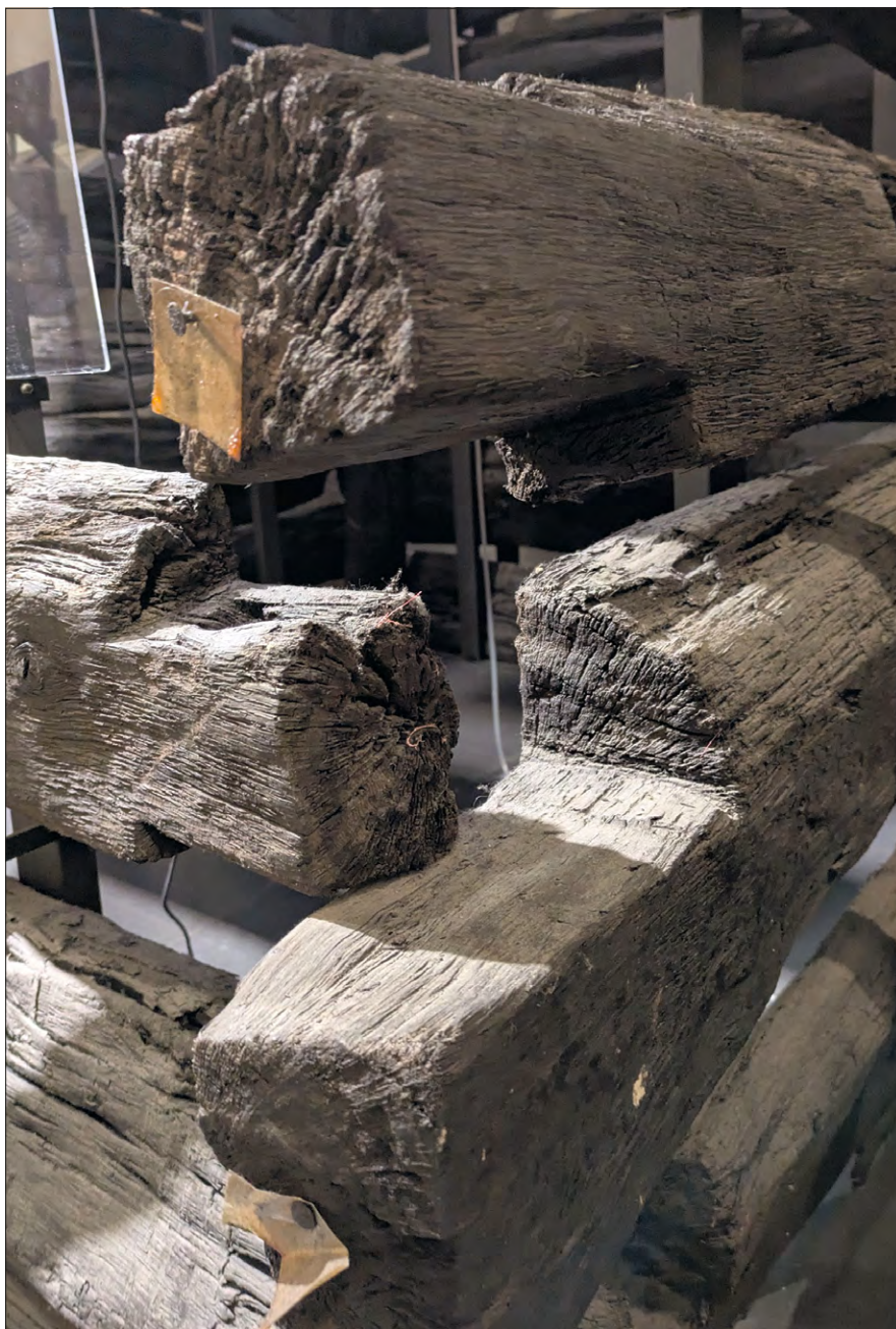
Fig. 5. Daps on elements of a well discovered in 2003 on Náměstí Svobody in Brno, reconstructed in the museum at Špilberk Castle in Brno, photo by R. Zdaniewicz.
