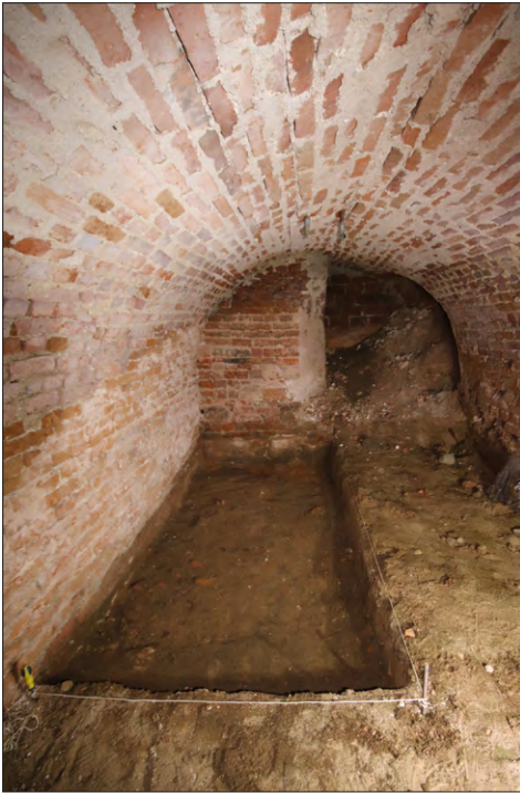
Fig. 5. The cleaned northern entrance hole with a visible excavation during exploration (photograph by M. Dobek).
