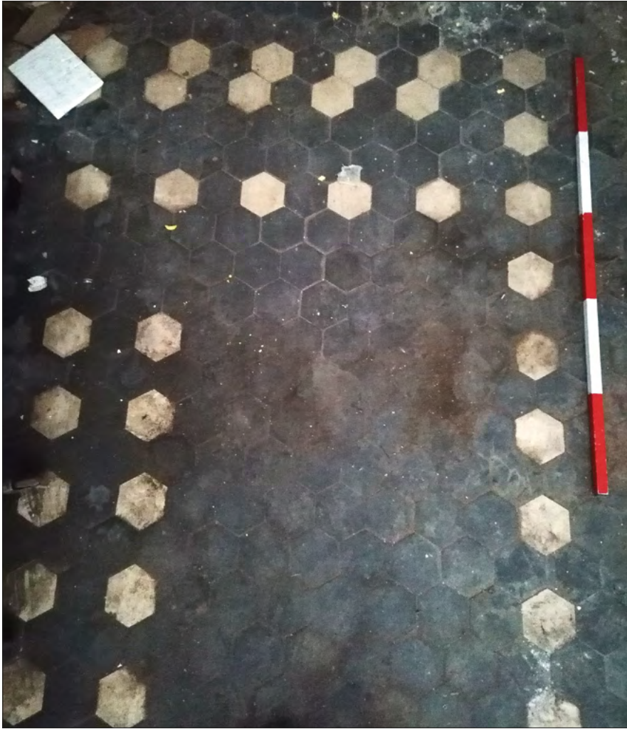
Fig. 17. 7 Anstadt Avenue, terracotta at the back of the school kitchen, the summer of 2019 (photograph by A. Majewska).
