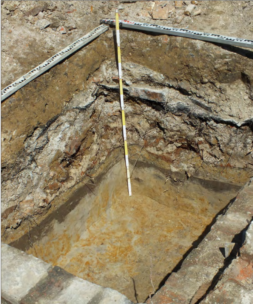
Fig. 6. The inside of block no. 6 (item 10), an exploratory excavation in the sw corner, E and N profile, a visible layer of the damaged levelling screed, insulation felt, and a base (photograph by W. Tabaszewski).
