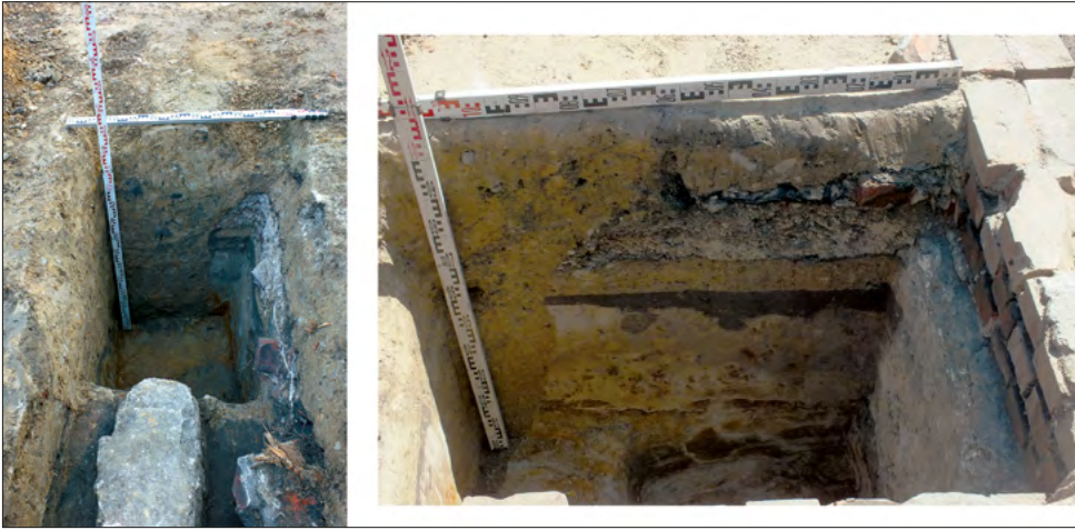
Fig. 14. An excavation at the S section of the W wall and at the NW corner of block no. 6 (item 10), in the N profile of both excavations one can see a secondary fill caused by the demolition of the foundations (photograph by W. Tabaszewski).
