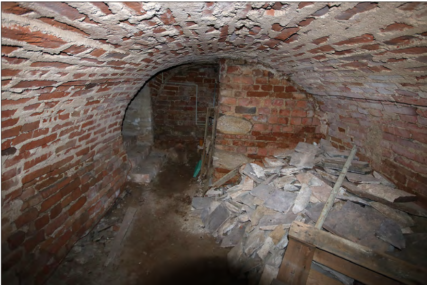
Fig. 2. Southern entrance to the crypt (photograph by J. Gawroński).
