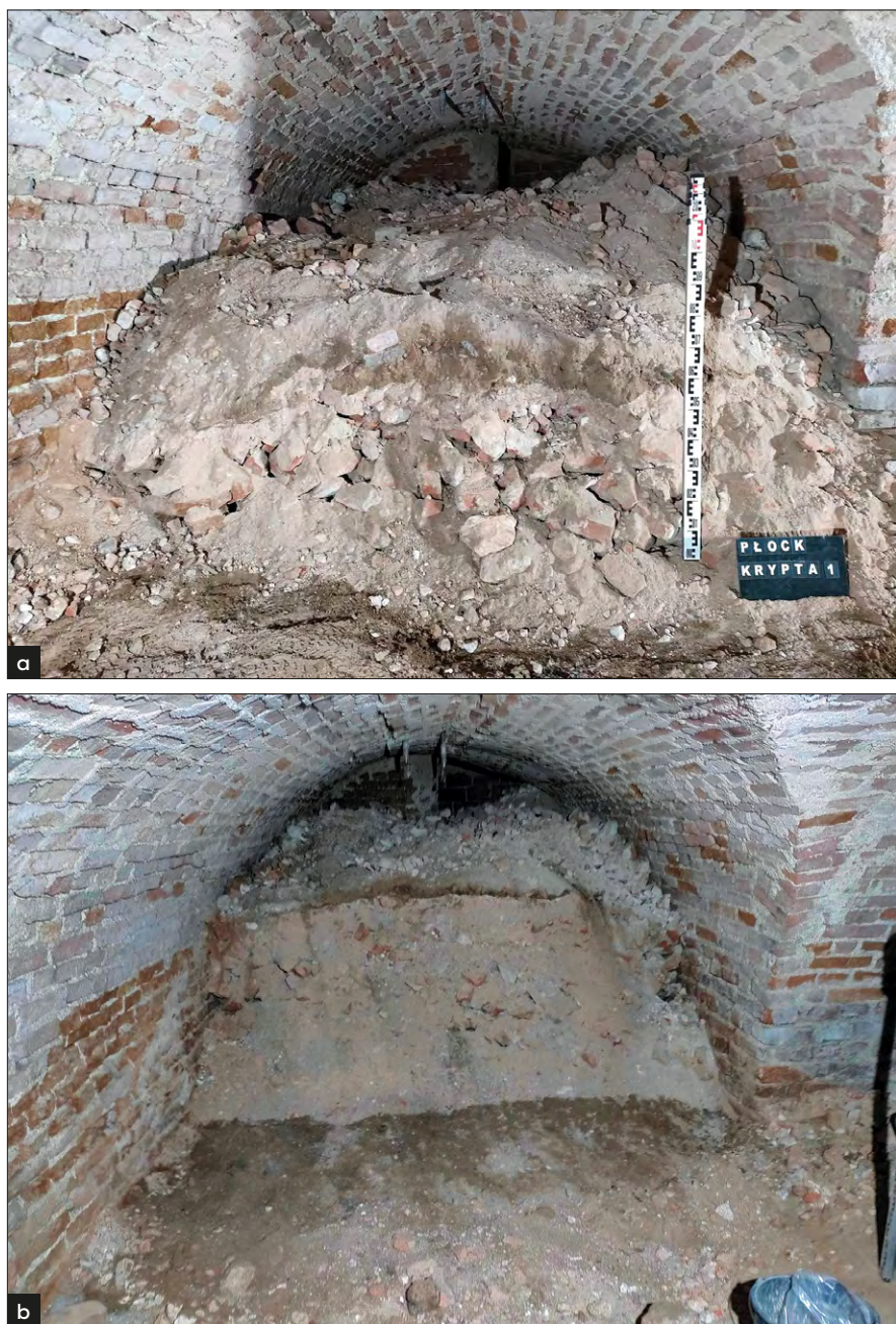
Fig. 3. Layers of the backfill during exploration: a – after uncovering layers of rubble with the remains of building material, b – during further exploration (photograph by K. Jasiak).
