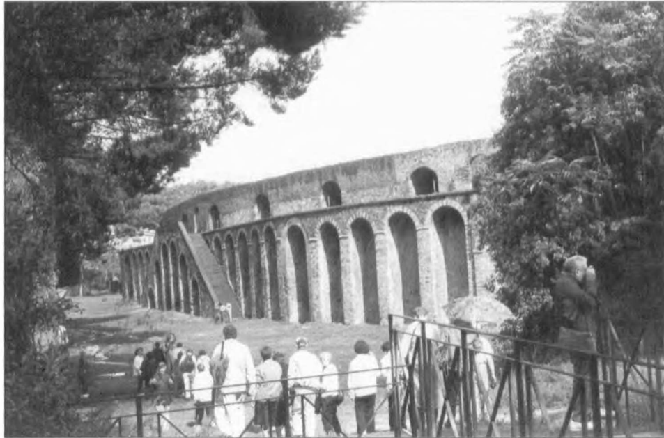
5. Pompeii, amphitheatre, first quarter of the 1 st c. BCE. Note the massive pilasters and vaults supporting the cavea (From: author's collection)
